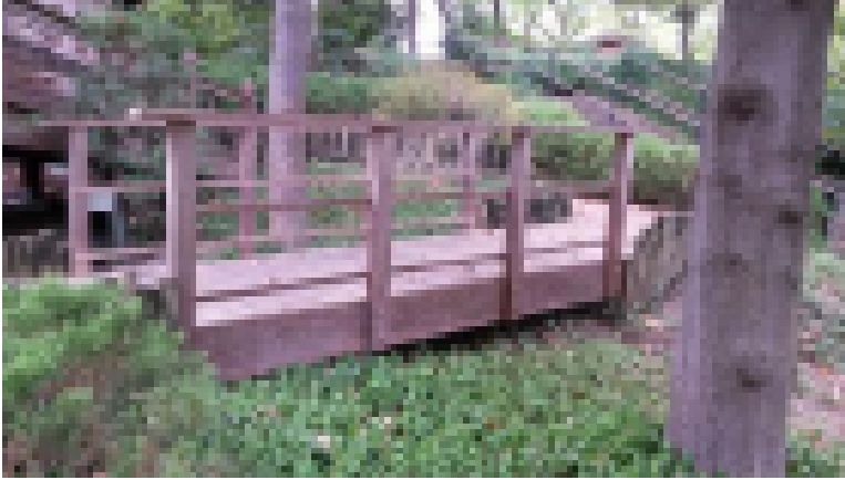
Wood Framed Bridge
