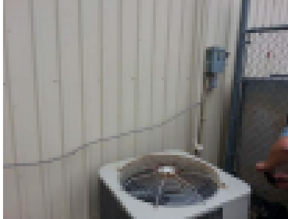
Exterior MC Cable Without Protection
