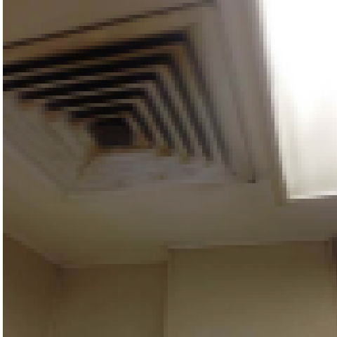
Rusted Air Device
