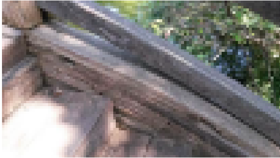
Deteriorated Beam
