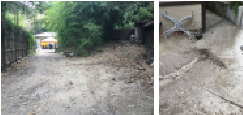
Existing Service Drive & Drainage Between Restaurant and Triplex Building
