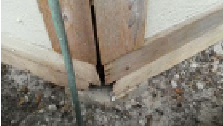
Trim in Disrepair
