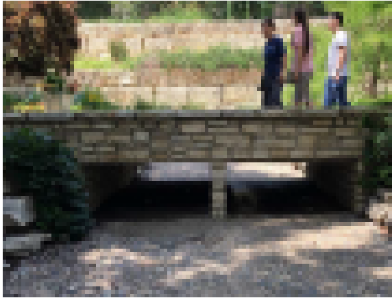
River Rock Swale Under Main Pathway
