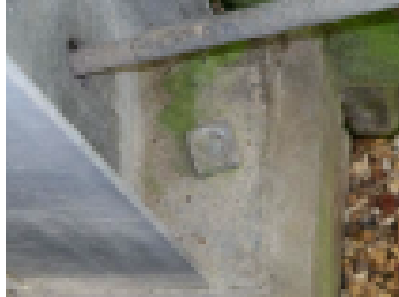
Plug Welded Anchor Bolt
