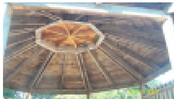
Trial Garden Pavilion Roof Framing
