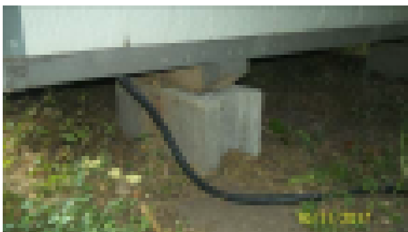
Shed on Concrete Blocks
