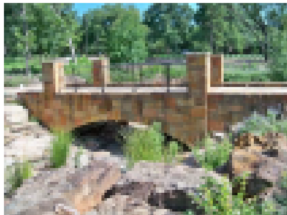
Stone-Clad Concrete Bridge
