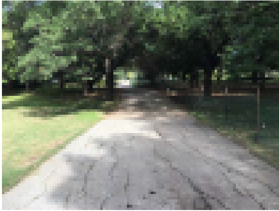
Asphalt Access Drive
