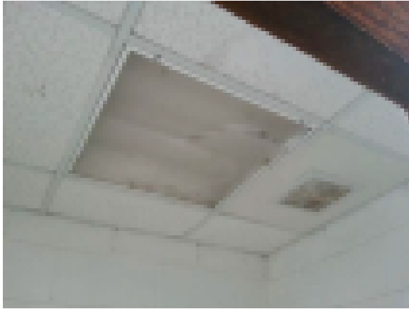
Lighting in Need of Replacement
