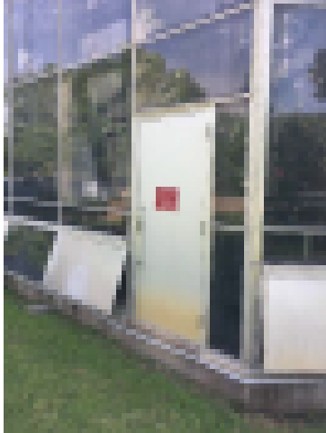
Emergency Exit (Exterior)
