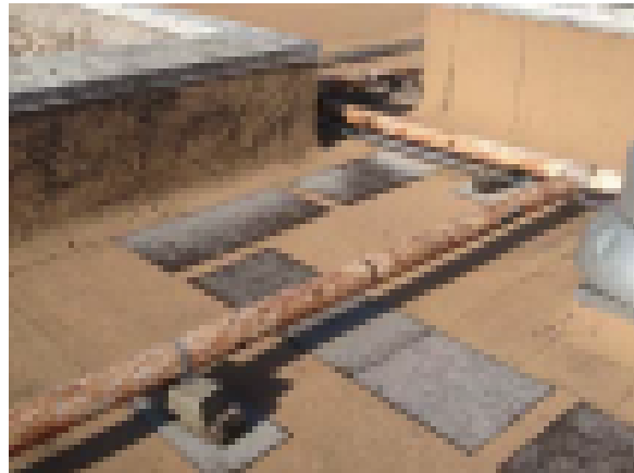
Rusted Natural Gas Piping on Roof
