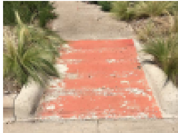
Pavement with Redwood Expansion Joints Ramp with Cracks and Peeling Paint
