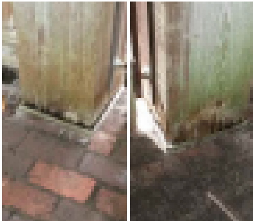
Post Deterioration
