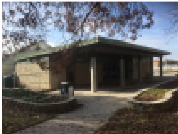
South Production Greenhouse Entry Canopy
