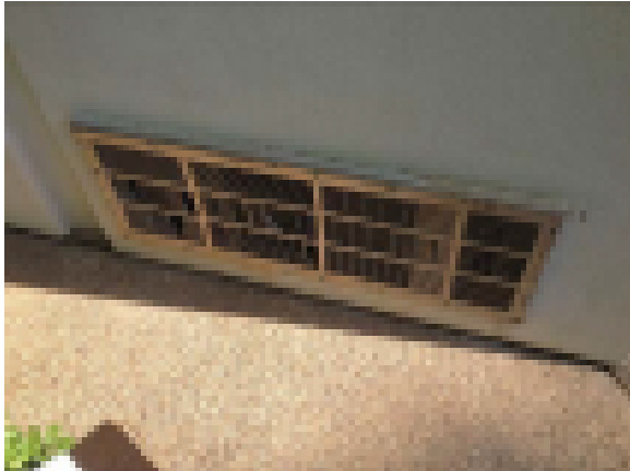
Damaged Unit Ventilator Grille
