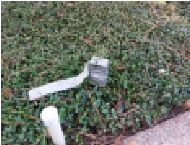
Damaged Receptacle
