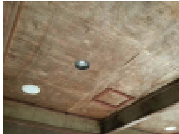
Downlights in need of upgrading
