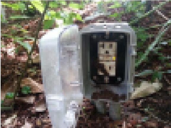
Damaged Receptacle
