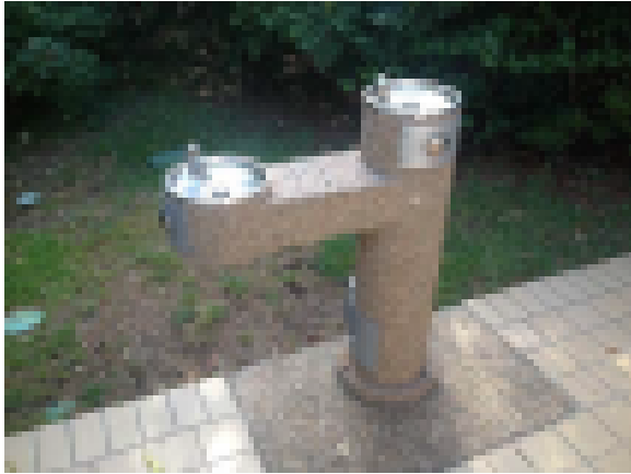
Exterior Mounted Drinking Fountain
