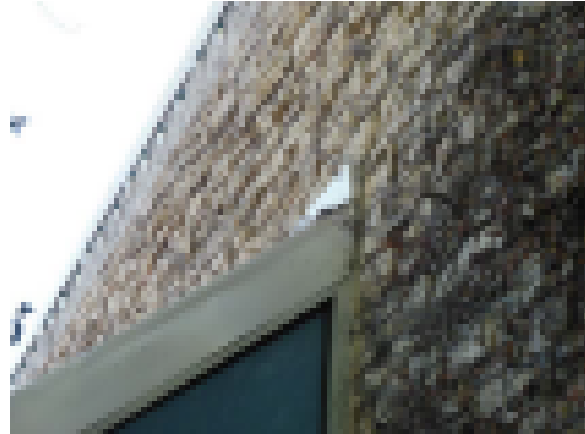
Flashing Damage
