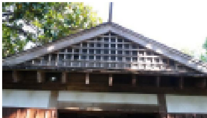
Wood Lattice Eave
