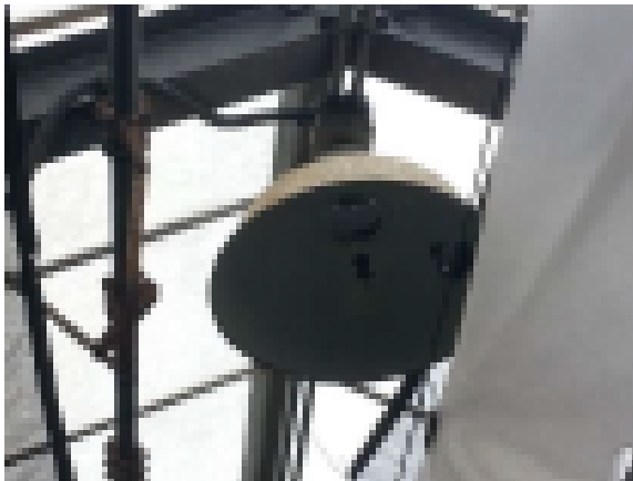
Example of Non-Operational Lighting Fixture
