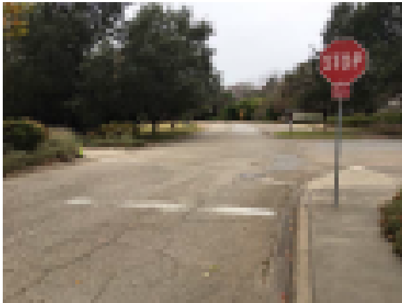
Worn Markings and Intersection Ramps
