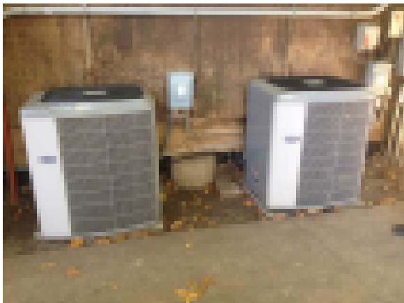
Existing two 5-ton condensers
