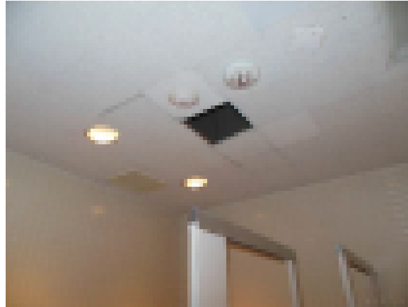
Missing and Damaged Ceiling Tiles
