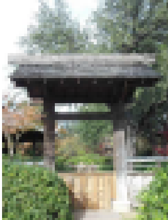
Exit Gate Structure
