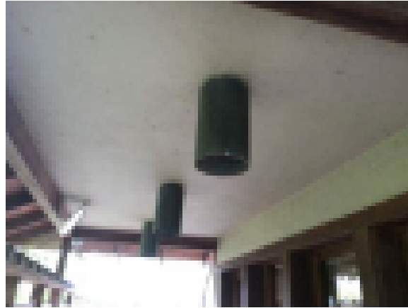
Exterior Cylinder Lights do not Light Adequately
