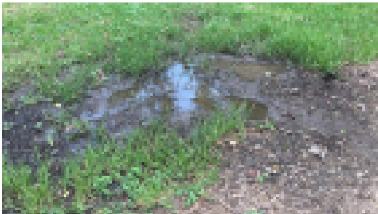
Standing Water / Muddy Areas Due to Wear and Lack of Positive Drainage
