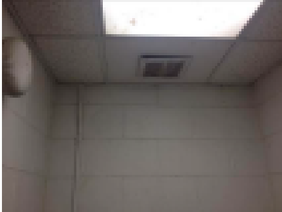
Exhaust Grille in Restroom
