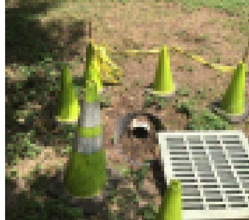
Localized Drainage Solutions
