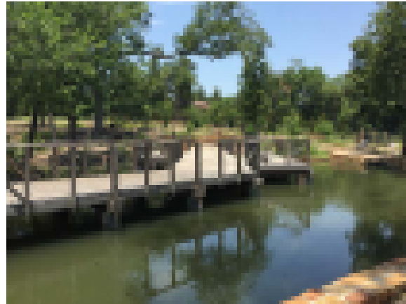
Wood Framed Boardwalk Over Pond #1
