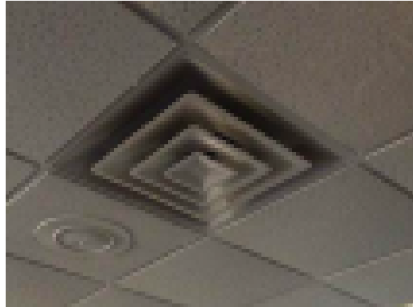
Rust on Ceiling Air Device
