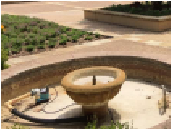
Water Feature in Disrepair
