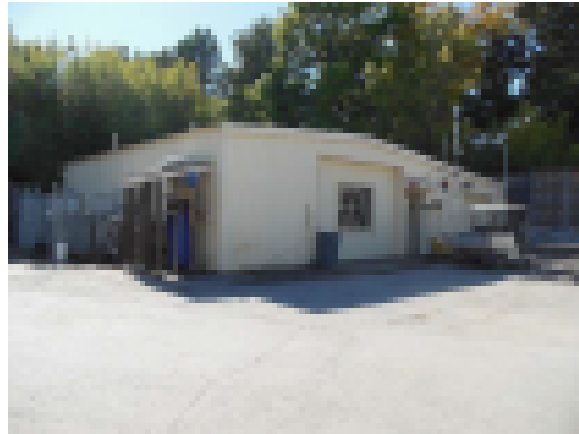
Break Room Building Exterior
