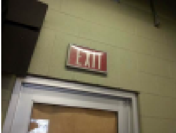
Non-illuminated exit sign
