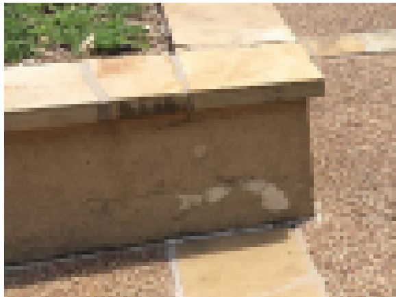
Stucco Veneer in Need of Repair
