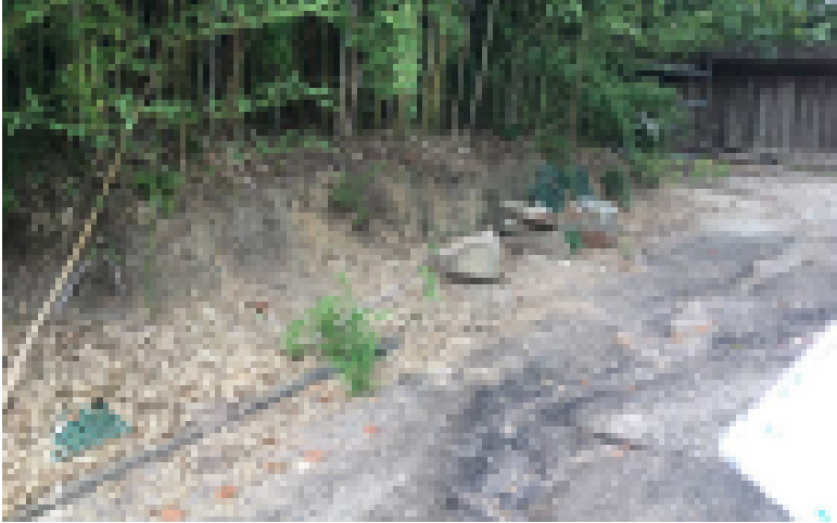
Slope Open to Erosion and Bamboo Growing with No Containment
