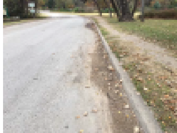
Sediment in Gutter and Worn Pedestrian Path
