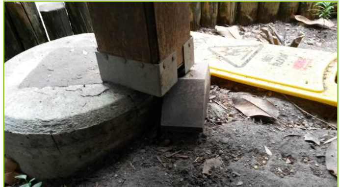
East Walkway & Ramp
